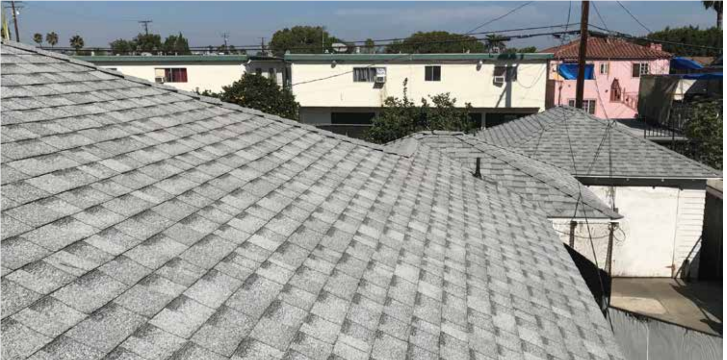
Single-family cool roof prototype that will be offered to Green Together project area residents free of charge. Photo credit: GRID Alternatives
